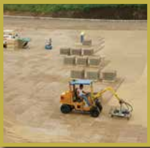
Mechanical installation, one pallet layer at a time, is an option for setting Renewable Pavers.
