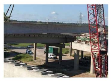
Additionally, throughout the corridor several improvements are taking place because portions of reinforcing steel bridge girders are starting to rust and deteriorate. These elements will be replaced and updated with concrete girders in addition to the traffic flow updates to serve the residents of St. Louis.
