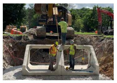
To avoid extended full road closure, delivery of the ready-to-install precast concrete components was optimized.
