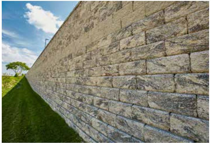
Available in several colors in Splitface and Rustic textures, Integrity units can be used to achieve any desired aesthetic. For this application, a band of complementary colored units were used to visually separate the massive retaining wall where it separates into two tiers, creating dimension. Wall caps also played an integral role in the project's dynamic design, as the caps define the wall's change in height as it slopes to the center of the tiers.
