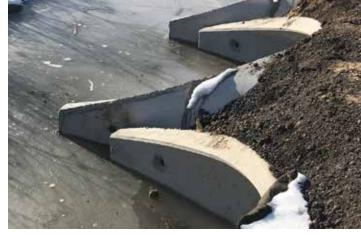
A representative from County Materials evaluated the site and recommended the installation of reinforced horizontal elliptical pipe. The elliptical shape allows for greater water flow in areas of shallow ground cover and flat terrain, while reinforced concrete pipe inherently has the longest service life of all culvert materials. The Village was pleased to approve this long-term solution.
