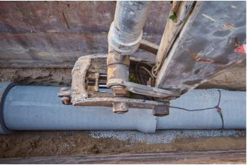
To accommodate the site's slope and the pipes' large size, sections of the system were installed 29 feet below ground, a depth only RCP can endure without excessive bedding and trench engineering.
