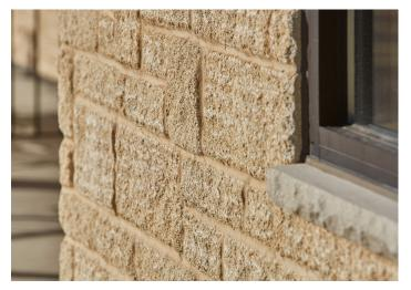
County Stone Masonry Units emulate the appearance of hand-hewn stone and offer the enhanced durability and cost-effectiveness of concrete masonry. Their high-strength concrete mix resists weathering and ensures longevity.
