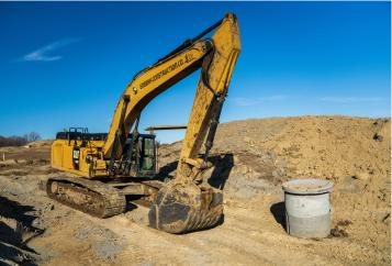
The City of Chaska specified concrete pipe and precast concrete structures for their longevity and low life cycle cost. Reinforced concrete pipe is a resilient material that strengthens with time and resists flotation to keep communities safe. Concrete pipe offers initial cost savings by requiring less bedding and compaction than alternative materials. These cost savings continue throughout the pipe's service life, which can reach up to 100 years.
