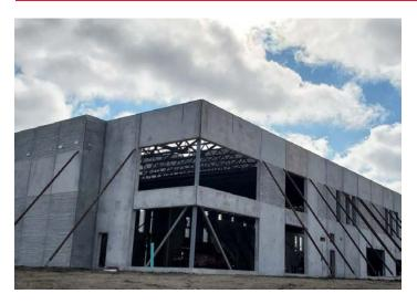
Architectural panels were produced with form liners that enhanced the aesthetic appeal of the activity center's façade. From reproducing textures found in nature, like wood grains and stacked rocks, to custom artistic patterns, form liners demonstrate the design flexibility of precast concrete.
