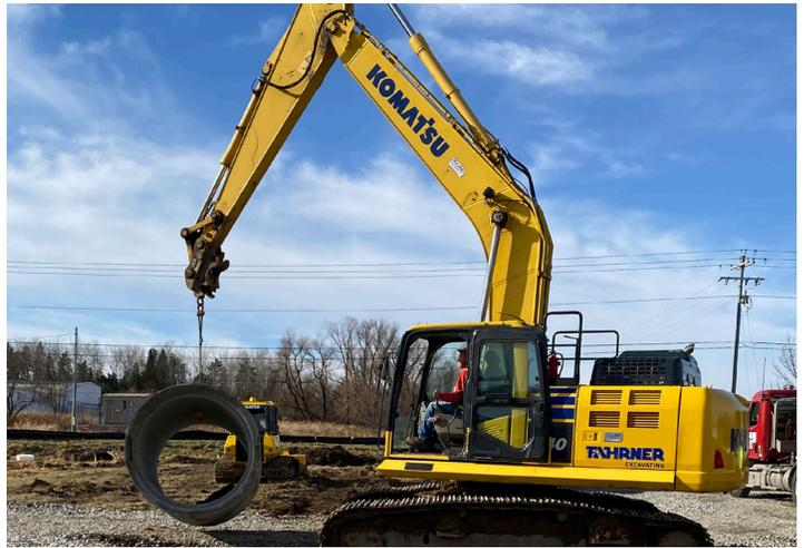
Kwik Trip relied on County Materials to supply 1,000 linear feet of concrete pipe in diameters from 15 to 60 inches. The storm water system was installed alongside the building and beneath its driveways.
