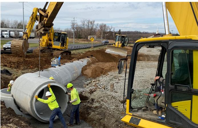
*Engineered and manufactured to optimize water flow and resist floatation, reinforced concrete pipe is a reliable storm water solution.*
