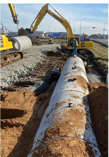
Engineered and manufactured to optimize water flow and resist floatation, reinforced concrete pipe is a reliable storm water solution.
