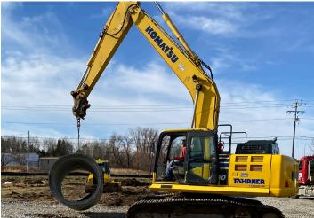
Kwik Trip relied on County Materials to supply 1,000 linear feet of concrete pipe in diameters from 15 to 60 inches. The storm water system was installed alongside the building and beneath its driveways.
