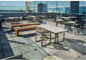
Installed using a pedestal system, the pavers form even joints that direct storm water and allow for proper drainage.
