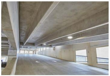
To seamlessly integrate the parking structure into its historic downtown surroundings, County Prestress manufactured beige spandrels, wall panels, and exterior columns and concrete brick infills. These components protect and visually enhance the structure.
