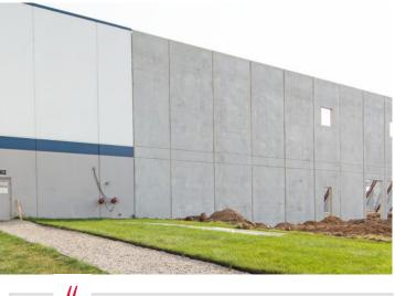
Comprised of two prestressed concrete panels that are separated by a layer of insulation, insulated sandwich walls are resilient and can maintain consistent indoor temperatures.
