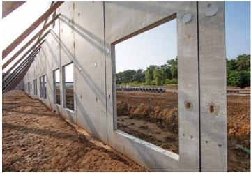
Insulated sandwich walls offer design flexibility and increase installation speed. County Prestress manufactured more than 150 insulated sandwich wall panels to complement Aisin Drivetrain's existing structure, emulating its characteristics. The panels were produced and cut to specification and arrived ready for erection, decreasing on-site costs and allowing earlier access for trades.
