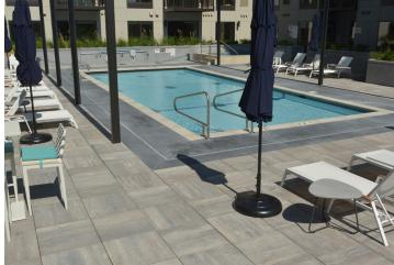
More than 10,000 SF of Skylands Concrete Deck Pavers were installed using pedestals that promote level, uniform paver placement on pitched and uneven surfaces. The pavers' even joints allow storm water to quickly pass into subfloor drainage, eliminating puddling, preventing property damage, and enhancing tenant enjoyment. Skylands pavers protect the roof membrane from years of exposure to weather and UV rays and can double its life expectancy.
