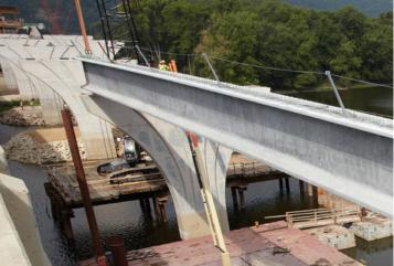
Each prestressed girder was manufactured to specification and ready to be installed upon delivery. The girders' height allowed for longer spans and required fewer support piers in the water, minimizing environmental impact and construction time.
