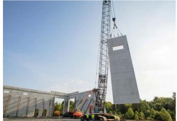
Insulated sandwich walls are comprised of two prestressed concrete panels that are separated by a thin layer of insulation. The panels' fabrication promotes consistent indoor temperatures and energy savings throughout their prolonged service life. Prestressed panels also resist weathering and forklift damage due to their exceptional strength and durability.
