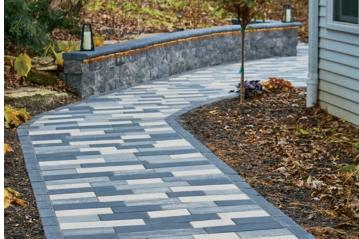
To create a level surface for the patio and provide additional seating, a 150 SF Tribute retaining wall and freestanding wall system was recommended. Two drains were built under the patio to move runoff away from the house.
