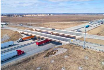
For highway infrastructure projects where limiting road closure time is a priority, prestressed girders offer many benefits over girders that are cast onsite. Prestressed girders arrive ready to install, accelerating the construction schedule. They also require less equipment to install, decreasing overall project costs.
