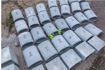
County Materials also supplied nearly 400 feet of concrete box culverts in spans of 12 feet by 5 feet to 10 feet by 6 feet. These precast concrete components function as short-span bridges and multi-barrel culverts and drains and are ideal for applications where other solutions are unable to provide adequate flow capacity.
