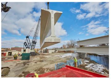
County Materials' Prestressed Bridge Girders were selected for their high-performance strength and durability. Prestressed girders can withstand heavy loads, ideal for the numerous motor vehicles that cross the bridge each day. Their inherent durability resists the elements, enduring freeze/thaw cycles during the winter months. Additionally, prestressed girders require minimal maintenance throughout their extended service life, reducing maintenance costs.
