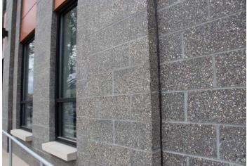
Premier Ultra Burnished units are integrally colored, and their surface is ground smooth to reveal natural aggregates for a result that replicates the look of hand-cut stone or granite for a fraction of the cost.
