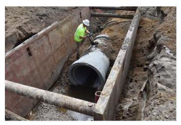
Where there are height or width restrictions, elliptical reinforced concrete pipe allows for higher flow capacities at shallower depths.
