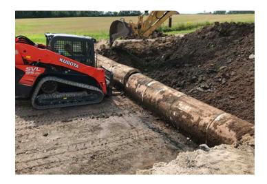
The project began by unearthing the existing concrete pipe. Crews exercised caution while removing the RCP, being careful not to disturb its end joints. Once above ground, the pipe was cleaned to look like new, and its joints were wrapped in filter fabric to prevent dirt from penetrating the drainage system. Once reinstalled, the end walls were set, concluding the two-day project.
