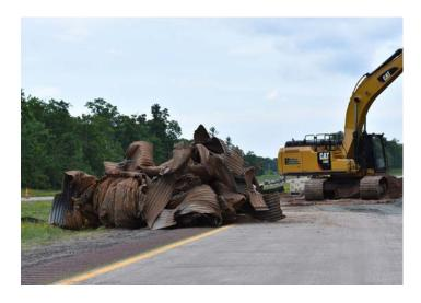
Construction crews prepared the site by removing the old storm water system, allowing the RCP to be installed upon delivery. County Materials' readily available concrete pipe and efficient delivery service allowed the accelerated construction schedule to be met.
