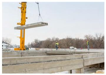
In addition to significant time and cost savings, ready-to-install prestressed hollowcore components from County Prestress offer high load capacity—key to spanning wider distances using fewer support columns—and high ratings for fire and sound transmission, making them an ideal solution for occupant safety and comfort.
