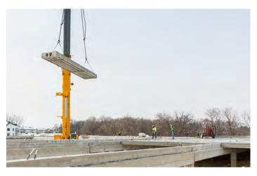
Faced with an aggressive construction schedule, project managers selected County Prestress' Hollowcore as the project's podium solution for underground parking due to short lead times and low life cycle cost.
