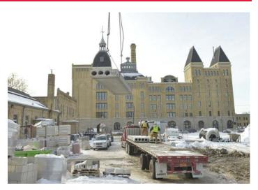
Ready-to-install components are manufactured to specification to accelerate the construction process. Production speed proved especially important for this project, which took place during a bitter Minnesota winter. By choosing prestressed components, which are manufactured in a climate controlled environment instead of being poured on-site, project leaders shaved several weeks from the construction schedule.
