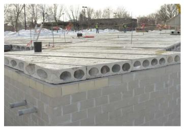
By choosing prestressed components, which are manufactured in a climate controlled environment instead of being poured on-site, project leaders shaved several weeks from the construction schedule.
