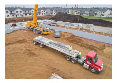
Ready-to-install prestressed components offer significant time and cost savings. County Prestress' Hollowcore and Columns and Beams are made to specification during production and arrive on site ready for installation. This process eliminates additional preparatory work, which reduces labor costs and site disturbance. With enhanced thermal properties, hollowcore provides high energy efficiency, leading to lower heating and cooling costs over its prolonged service life.
