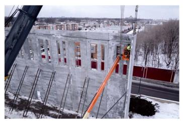
The concrete wall panels' thermal mass effectively stores and releases heat, resulting in an energyefficient structure that will save money throughout the project's service life.
