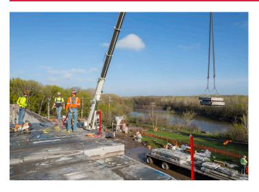
Once installed, hollowcore provides an instant work deck, which helps crews maintain construction schedules and reduce lost time. For this project, the erector set almost 60,000 square feet of hollowcore in just three weeks, allowing early access to the site for other trades.
