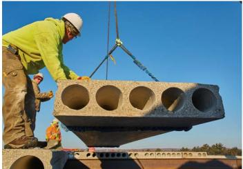
County Prestress' hollowcore offers speed of installation and structural benefits. Hollowcore is manufactured to specification and prepared to be installed upon delivery, optimizing construction timelines. Hollowcore can be installed year-round. This facility was constructed during the winter months to prepare for the growing season ahead. Hollowcore provided a long-lasting storage solution with minimal disruption to agricultural operations.
