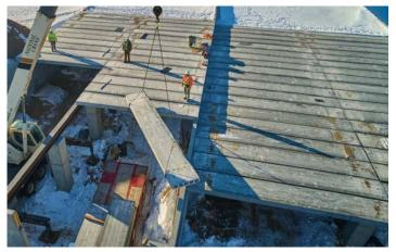
Hollowcore was used for its high-performance strength, allowing long spans to be constructed without the need for additional columns, providing greater functionality for the root drying facility.
