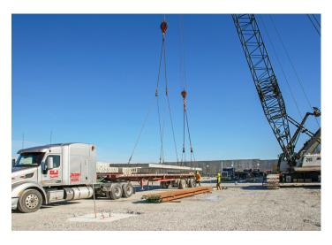
County Prestress' Insulated Sandwich Walls are manufactured to specification and arrive on site ready for erection. Prestressed panels promote ease and speed of installation, meeting tight construction schedules and allowing trades earlier access.
