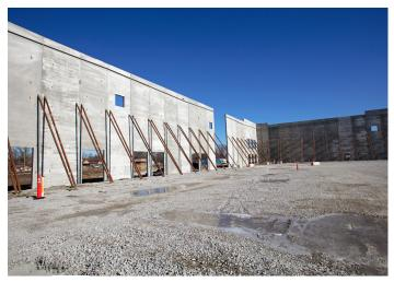
County Prestress' Insulated Sandwich Walls are manufactured to specification and arrive on site ready for erection.
