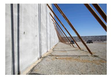
Within two weeks, 130 panels containing 66,550 SF of prestressed concrete were installed. Insulated sandwich wall panels can be installed in most weather conditions and since they are manufactured by County Prestress offsite, construction times can be shortened.
