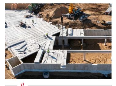
Once installed, the planks serve as an instant, stable work deck to keep sites cleaner and promote efficiency.
