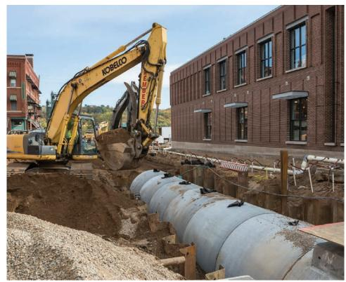
Concrete pipe maintains structural integrity over a service life of 70 to 100 years.
