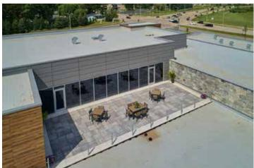
Skylands Concrete Deck Pavers are installed on a pedestal system that is designed to transform underutilized spaces. These systems accommodate a range of slopes for diverse applications. Using a pedestal system, pavers are installed evenly to promote proper drainage through joints, preventing puddling and improving pedestrian safety. Once installed, the complete system protects the roof below from seasonal elements while ensuring easy maintenance access.
