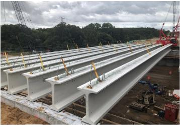
WisDOT relied on County Materials to manufacture and deliver 16 prestressed girders within the accelerated timeline, utilizing two facilities to maximize production.
