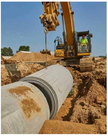
The low life cycle costs and longevity of RCP made it a viable option for this large-scale project.
