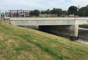
Structural components were placed piece-by-piece during the simultaneous excavation of the underpass and construction of the bridge. Arriving on site ready for installation and immediate use, precast pier caps were essential in maintaining railway operations as construction proceeded below. Once the precast and steel structure was erected, prestressed fascia girders were installed on its exterior to protect against over-height vehicle collisions and prevent disruptive reconstruction.
