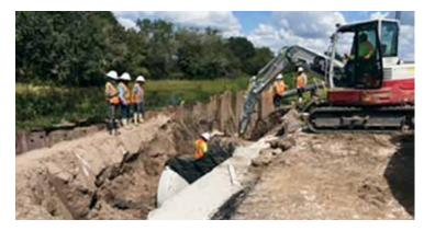
Contractors worked around the clock to meet the deadline. When they first arrived on site, they saw that much of the soil surrounding the drainage pipe had washed out, causing the weight of the road to crush the corrugated steel pipe that was originally installed. To prevent another road collapse in the swampy area, Florida Safety Contractors chose reinforced concrete pipe manufactured by County Materials in Astatula, FL.
