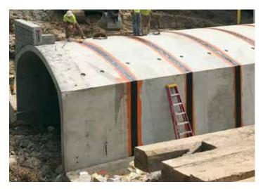
Aesthetics were also an important consideration, as the project was located in a growing part of the city. Unlike traditional options, such as standard culverts, the ArchCast Precast Bridge System offers enhanced aesthetics through its decorative facing that emulates natural stone. This design element elevates the project's overall appearance without additional labor.
