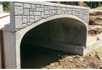
Valuable time was saved on site, as the ArchCast units were manufactured to specified sizes and arrived ready to be installed.
