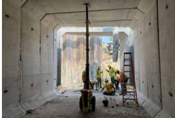
Engineered and manufactured to withstand harsh underground environments, precast box culverts proved as an ideal solution for this hydroelectric facility. County Materials manufactured nearly 140 16'x14' precast box culvert sections for the facility. Each precast component was manufactured to specifications, eliminating the need for on-site cutting and additional preparations. This afforded the project the efficiency needed to meet its tight construction schedule.
