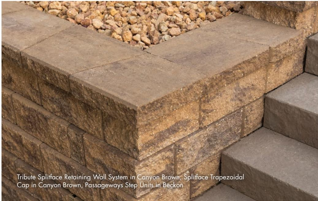
Tribute Splitface Retaining Wall System in Canyon Brown, Splitface Trapezoidal Cap in Canyon Brown, Passageways Step Units in Beckon
