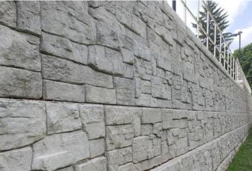
In addition to structural benefits, Rib Rock Landscape Block offers time and costs savings. The oversized units are capable of covering twice the area in less time with the use of smaller crews. Rib Rock installation is straightforward by utilizing equipment to expedite the process and place the heavy units. Over 5,700 SF of Rib Rock in Dry Stack texture was used to transform this property to reach its full potential.
