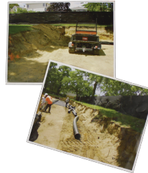
Photos of future retaining wall site
