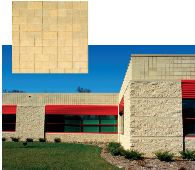
Figure 1 – Examples of SMOOTH Colored CMU Walls
